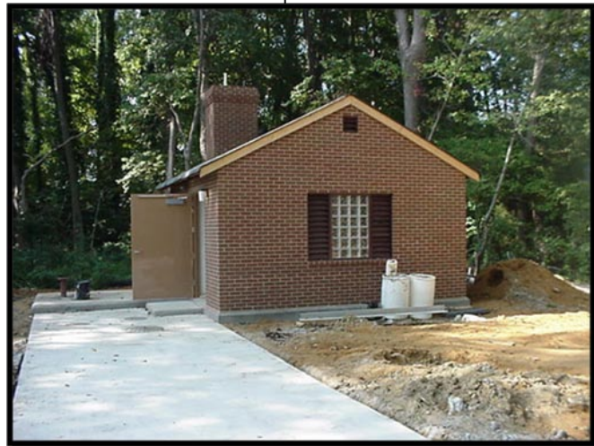
Dare Heights Sewage Pump Station, Shutters are really louvers.
