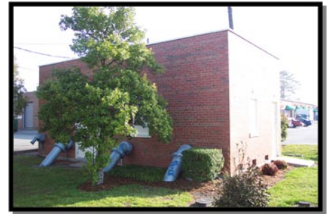
Masonry buildings were evaluated for resistance to Category II hurricane winds.
