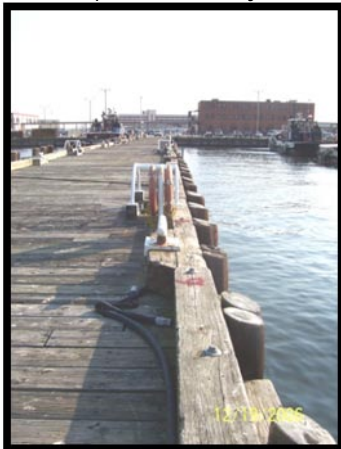
Existing Pier F, Deck
