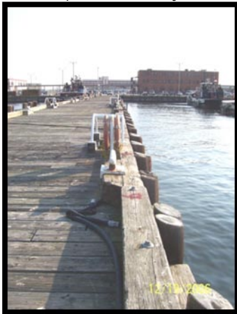
Existing Pier F, Deck
